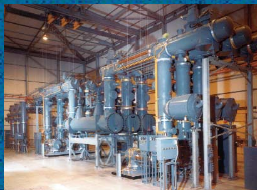
Compressed air dryers
